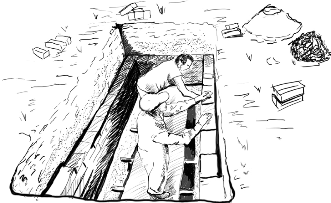
Figure 13: Pit lining with bricks
