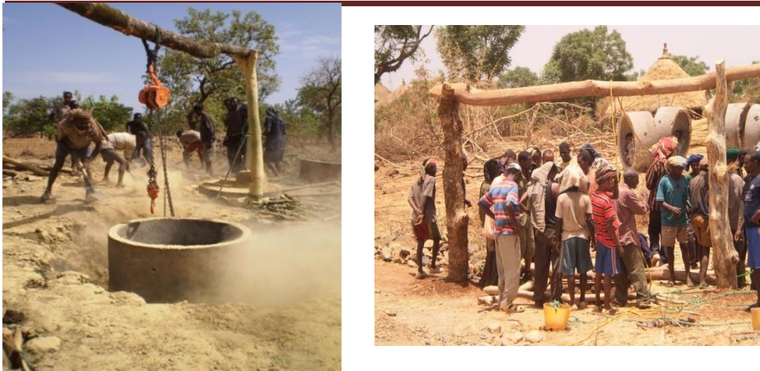
Figure 15: Community contributing free labor for well construction
