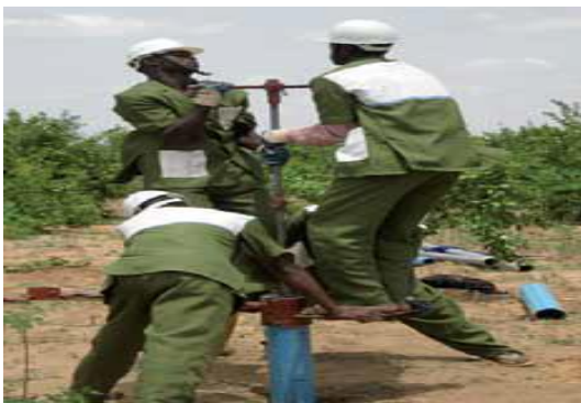
Hand Auger Manual drilling (3) & percussion (4)
