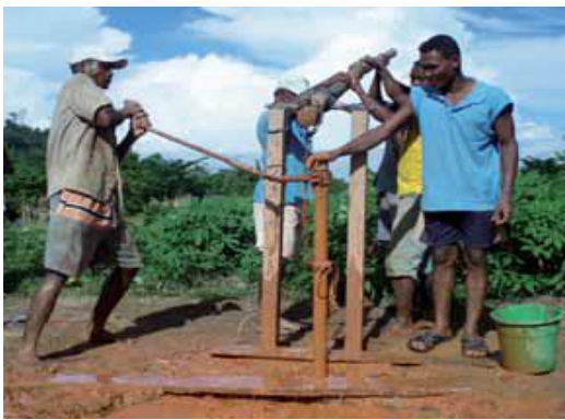
Sludging (1) type of manual drilling & jetting (2)
