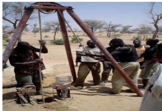
Hand Auger Manual drilling (3) & percussion (4)
