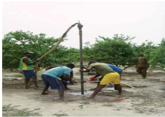
Sludging (1) type of manual drilling & jetting (2)
