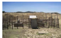
Tap stand connected to spring
