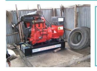
A new generator but already cracks are appearing in the base and the location of the generator is not well protected.
